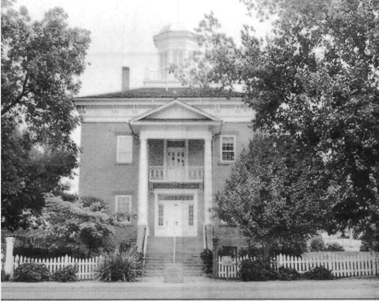
Figure 60: Washington County Courthouse
